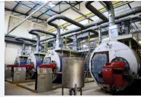
Energy recovery from residual energy in power stations
