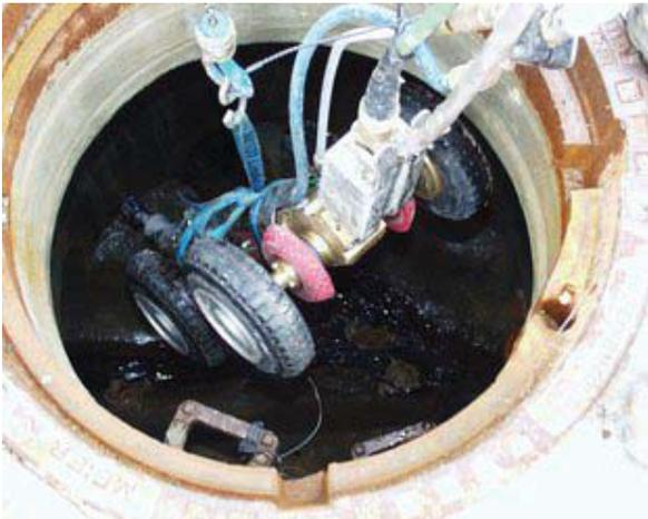
applications technician Sven Menzel of GM-San UG. And he stressed: "With the F170 and the new DEPRAG air motor the work involved in opening the branch-outs is much faster."
